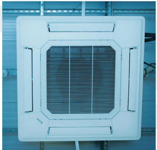
Please be aware that your systems may go into defrost mode occasionally during the day. At this point the indoor unit will appear to stop heating. This is normal operation and it should last between 5 and 10 minutes, at this point the outdoor condenser unit will be defrosting. Once defrosted the indoor unit will start again and continue to heat.
